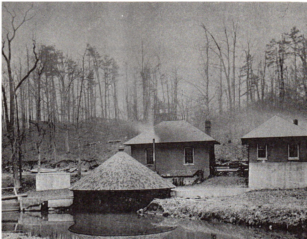
Takoma Park Filtration Plant
