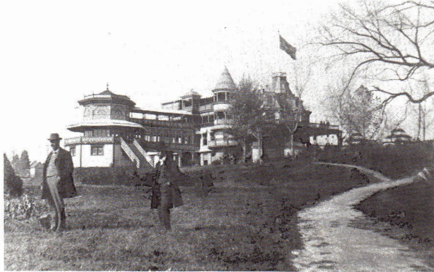
Rear View of the Cabin John Bridge Hotel Showing the Stained Glass Housing for the Orchestration
