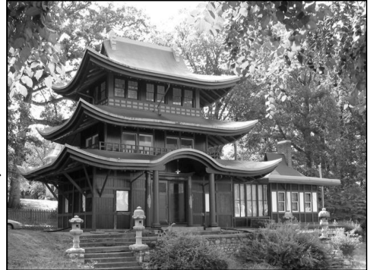
Save Our Seminary restored the exterior of the Pagoda sorority house to show what could be done with other buildings on the campus.
